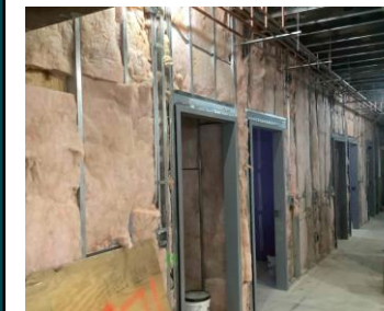
In-wall soundproofing
