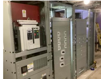
Main electrical gear partially assembled
