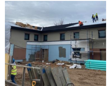
Installation of metal roofing
