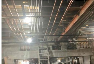
Plumbing piping installation
