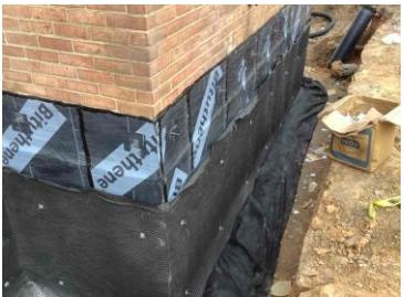
Waterproofing foundations
