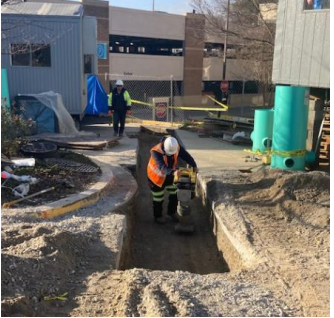
Backfilling site utilities
