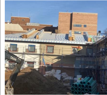
Roof waterproofing installed
