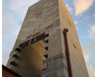
Constructing elevator shaft
