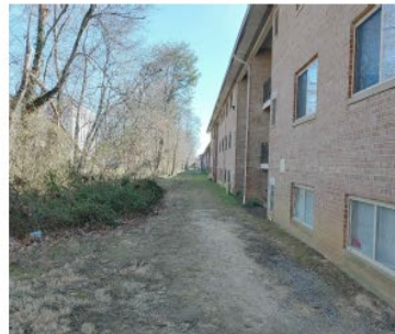
REAR OF BUILDING #1 SERVBACK AND UTILITY AREA
