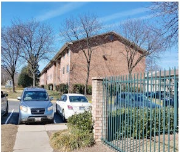
END OF BUILDING #2 TYPICAL BUILDING STREETSCAPE
