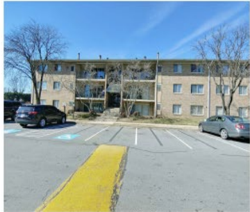
BUILDING #3 TYPICAL BUILDING BLOCK VIEW
