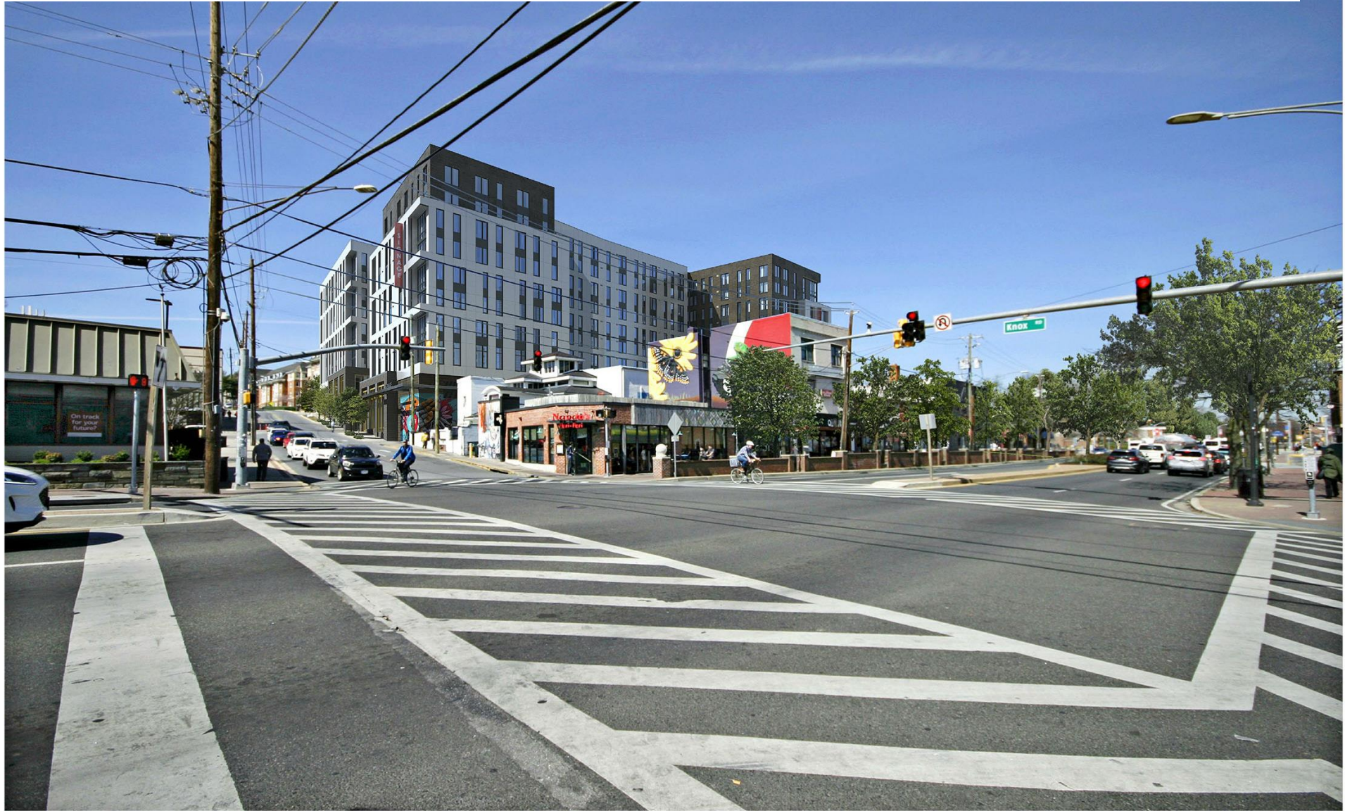
3 - VIEW FROM THE CORNER OF US ROUTE 1 (BALTIMORE AVE) AND KNOX ROAD LOOKING NORTHWEST
