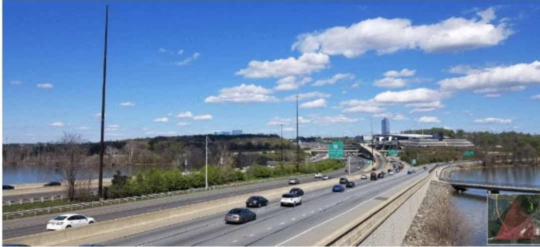
BELTWAY OVERPASS TOWARDS DEVELOPMENT
