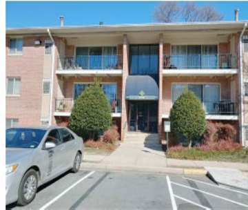
BUILDING #1 TYPICAL 2.5 - 3 STORY BUILDING
