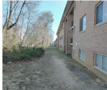
REAR OF BUILDING #1 SETBACK AND UTILITY AREA
