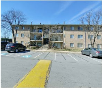
BUILDING #3 TYPICAL BUILDING FACADE VIEW
