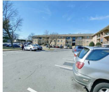
BUILDING #3 TYPICAL BUILDING FACADE & CONNECTIVITY
