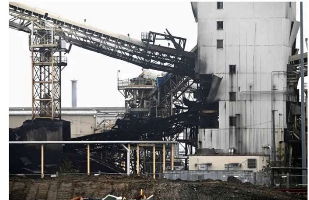
Damage from the explosion is seen on the coal transfer tower of the CSX Curtis Bay Pier.
