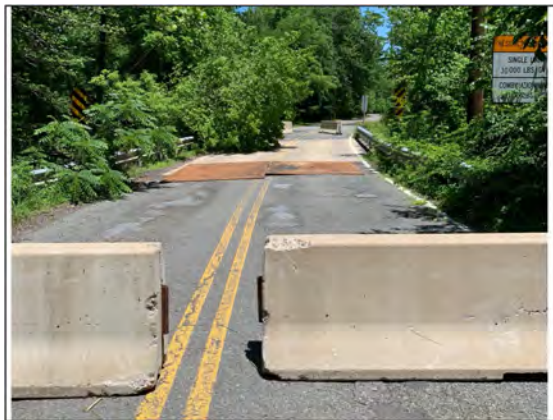
Steel Plates Over 4' x 3' x 8'deep sink hole
