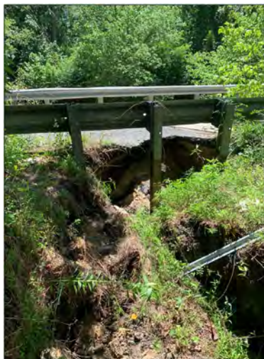
Slope failure next to culvert
