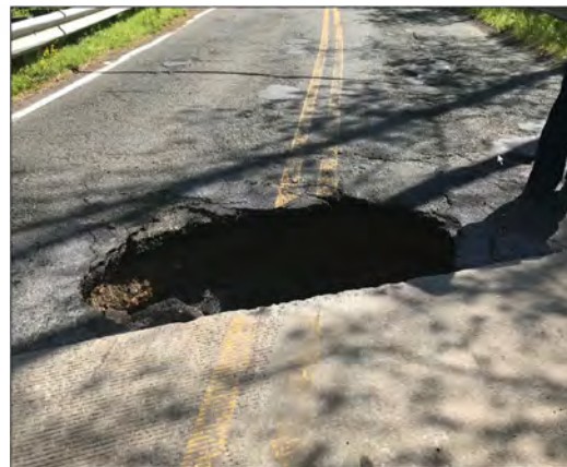
Hole in Road Prior to Being Covered by Steel Plate
